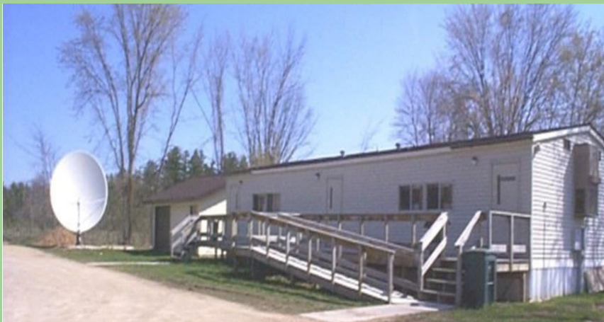
Above: Old Main - First building on the CMN Main Campus. It's still there today!
