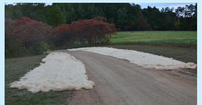
Finished product, planting grass to regrow in the disturbed area
