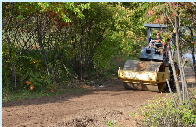
Rolling and flattening the drive way
