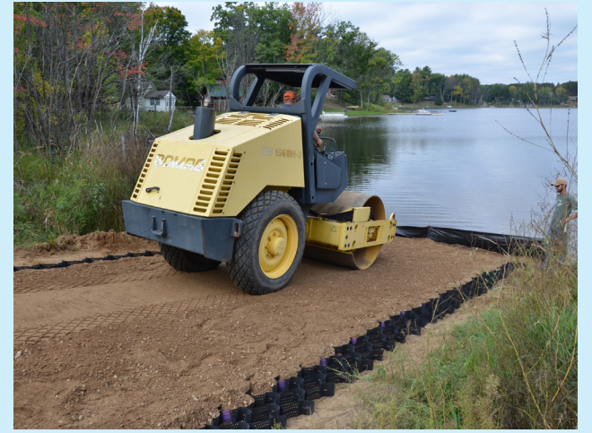
The roller packing down the gravel
