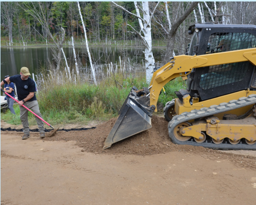
Filling the sides and and low points
