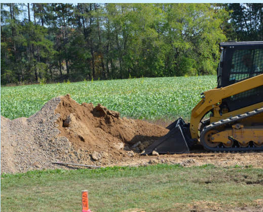
Skid steer picking up gravel to fill the driveway
