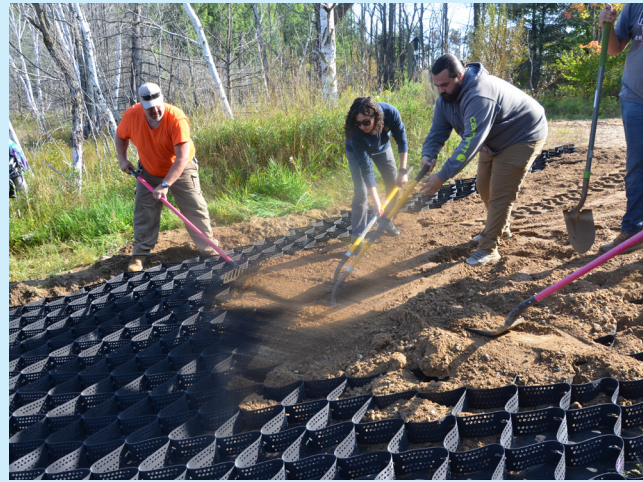
The black Envirogrid material being filled with Gravel
