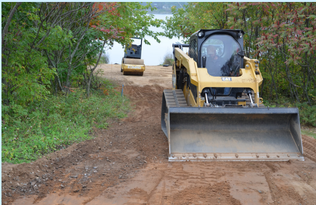
Starting to work on the driveway
