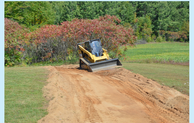
Diggin out the corner to improve turning and water run off
