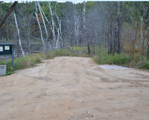
Rolling and flattening above the boat launch
