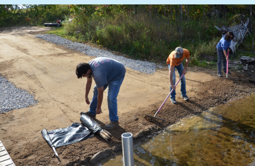
Removing silt fence from water
