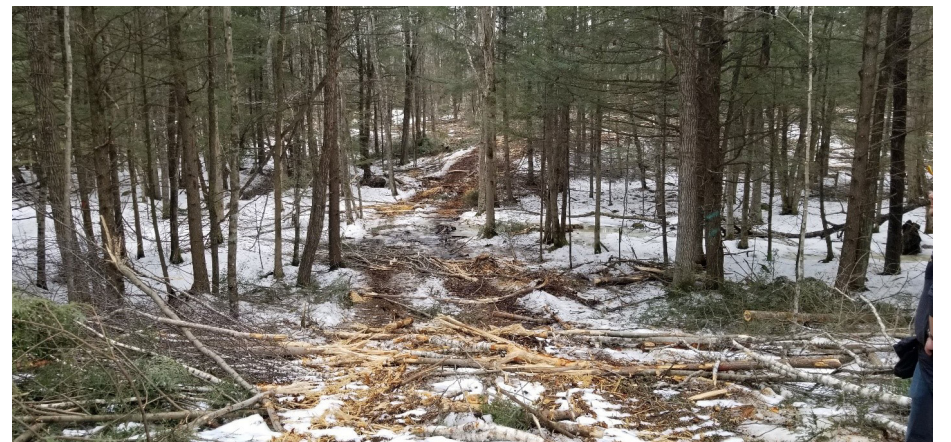
Wetland crossing where slash was laid down during operations and removed once completed.
