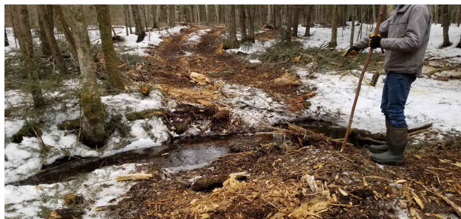
Great looking stream crossing; slash and timber mats were used during operations and removed when done.
